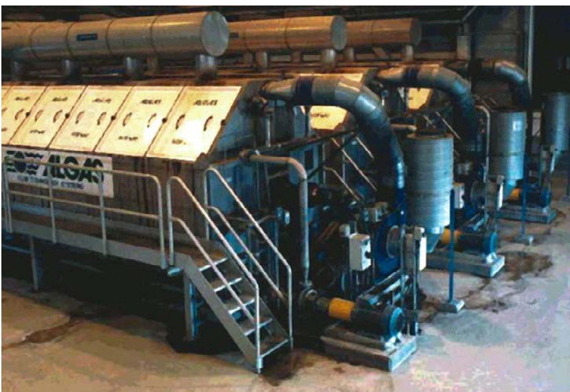
No sedimentation basins – just compact Algas Microfilters for primary effluent treatment.
